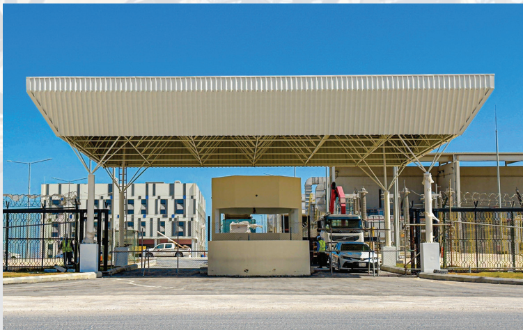
SWCC Security Gate Sunshade, Jubail
