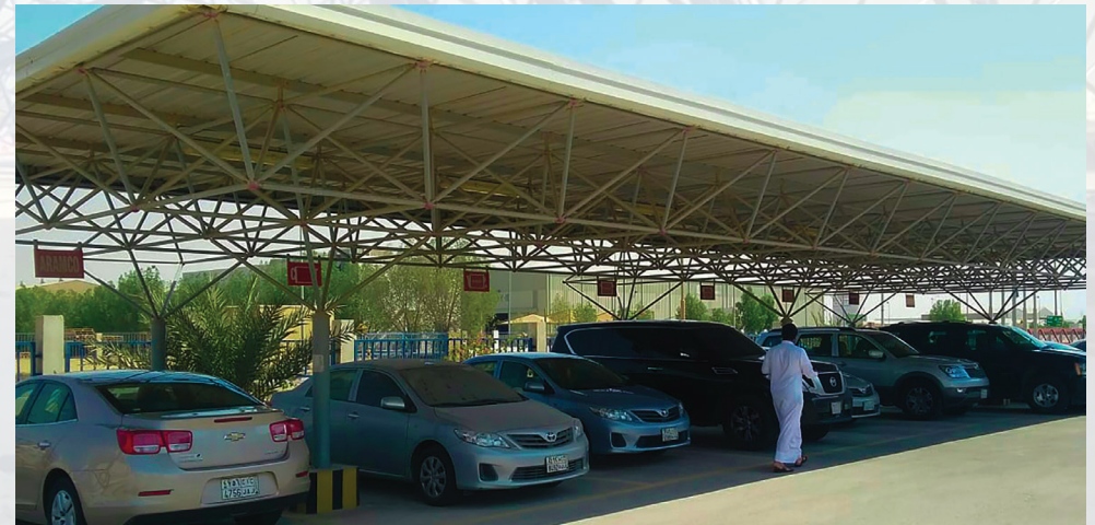
Car Parking Shelter
