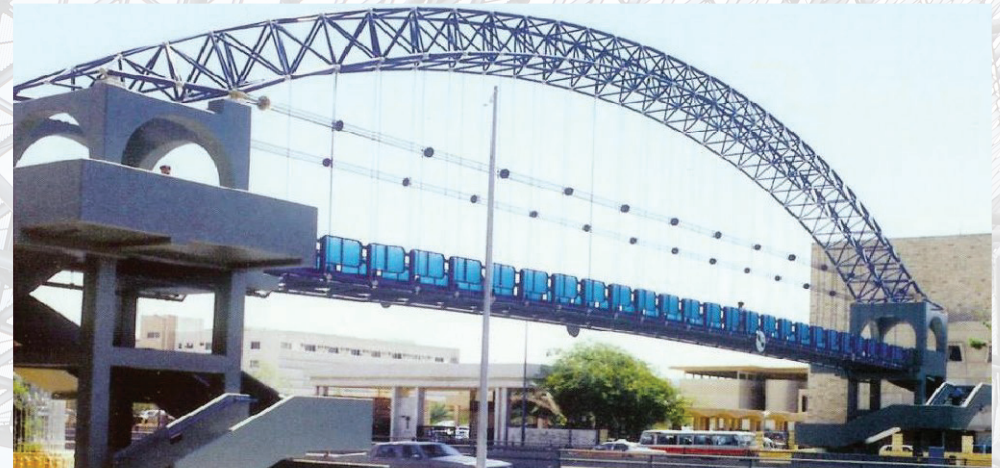
Pedestrian Suspended Arch Bridge
