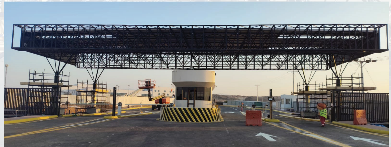
NEOM Community 2 Security Gate Sunshade
